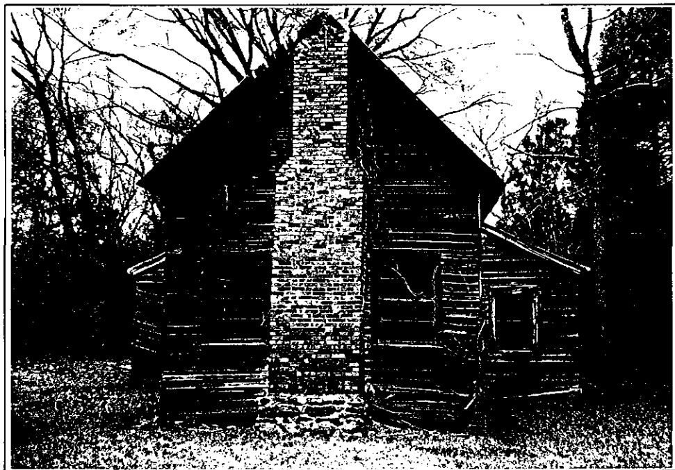
McCormick Farmstead. 1821 House, South Facade of c.1890's Addition.
