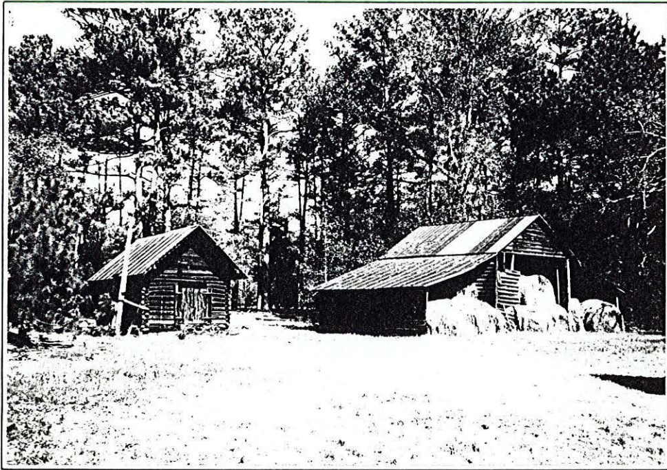
McCormick Farmstead. Northernmost Crib and Barn from the South.
