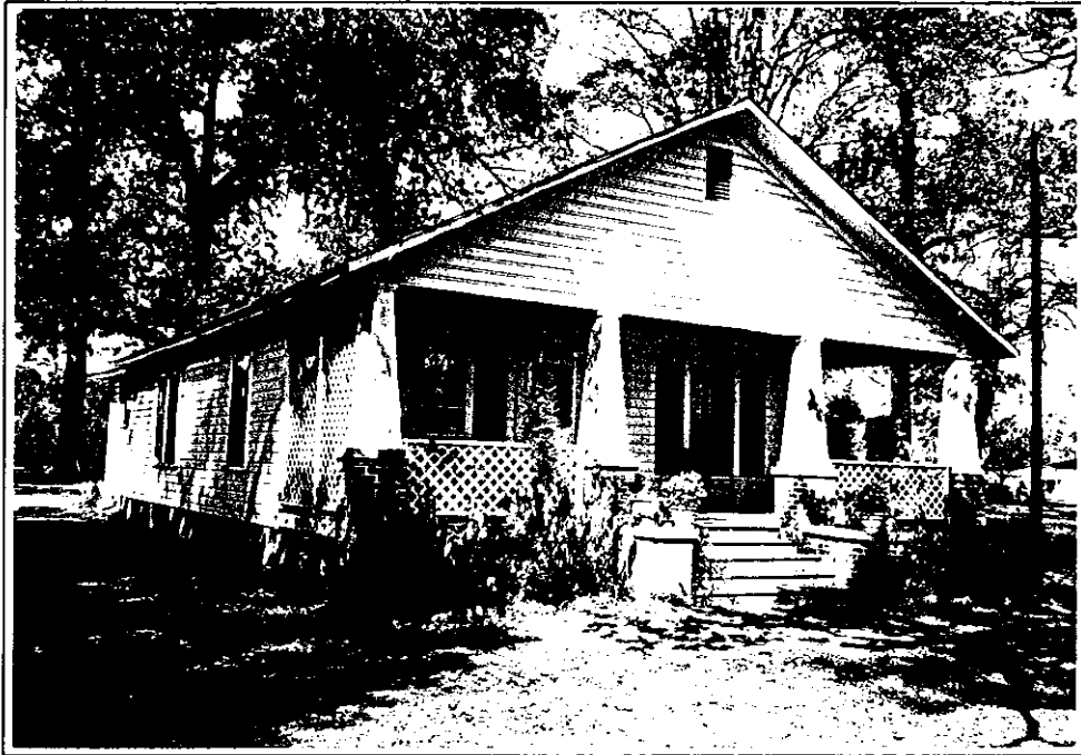
Early Twentieth Century Craftsman-Style Suburban House, North Side of SR 1451.
