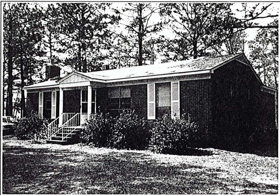
McCormick Farmstead. 1958 House from the North.
